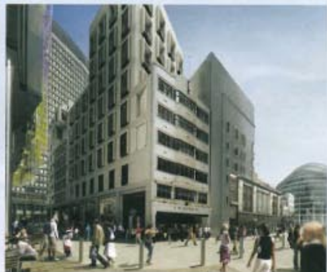
The north elevation incorporates a retained, listed facade.
