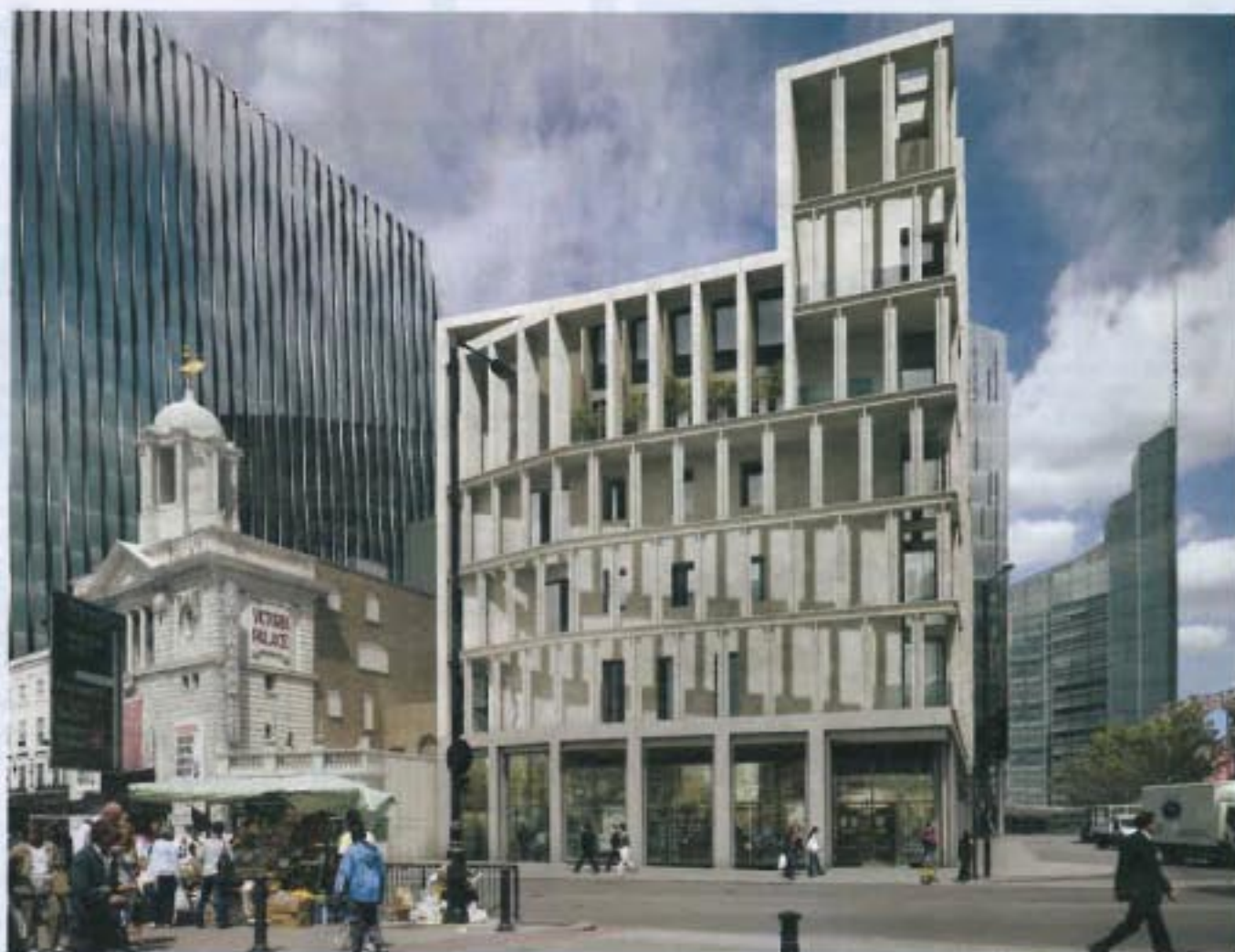
The library, on the south end of the development, addresses Victoria Street.
